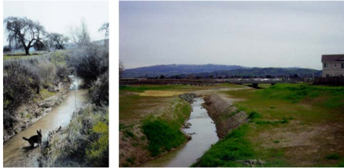
Figure 2. Pre-restoration incised channel (left) and post-restoration compound channel (right) in Tassajara Creek restoration project reach.
