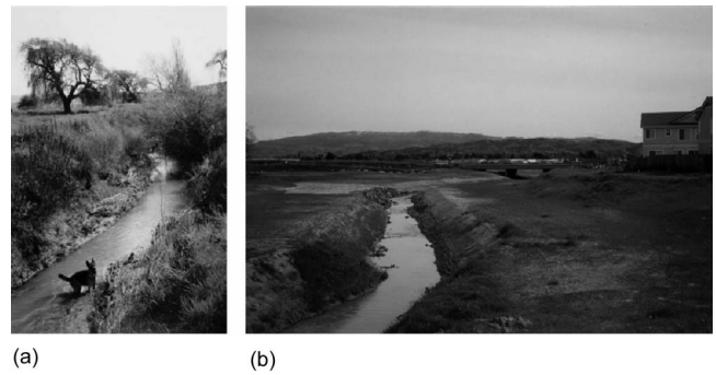
Fig. 2. (a) Prerestoration incised channel; (b) postrestoration compound channel immediately following construction in Tassajara Creek restoration project
